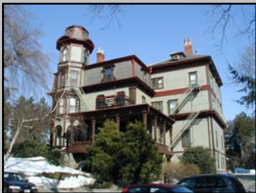
990 Centre Street Historic Renovation
