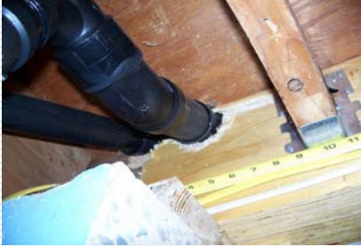
JSL Engineering, Inc. Inspecting the Structure System, ASHI-NE 6 th Annual Conference
