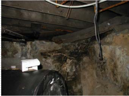
JSL Engineering, Inc. Inspecting the Structure System, ASHI-NE 6 th Annual Conference
