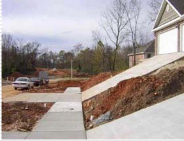
JSL Engineering, Inc. Inspecting the Structure System, ASHI-NE 6 th Annual Conference
