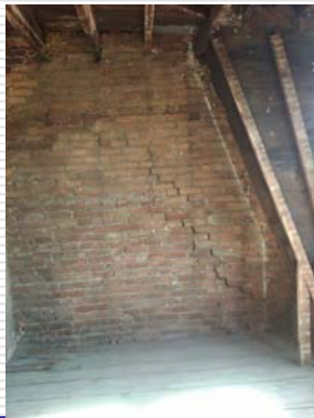
JSL Engineering, Inc. Inspecting the Structure System, ASHI-NE 6 th Annual Conference
